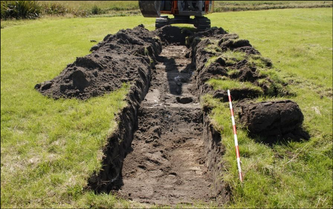
Plate 12 View of pre-development test trench excavated through approach road
