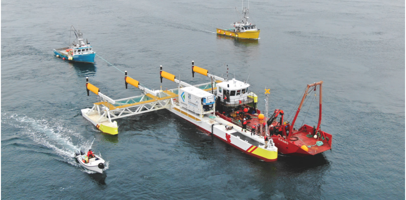
SMEC Plat-I Installation, Grand Passage, Nova Scotia, Canada Courtesy: Sustainable Marine Energy (Canada) Ltd. (SMEC)
