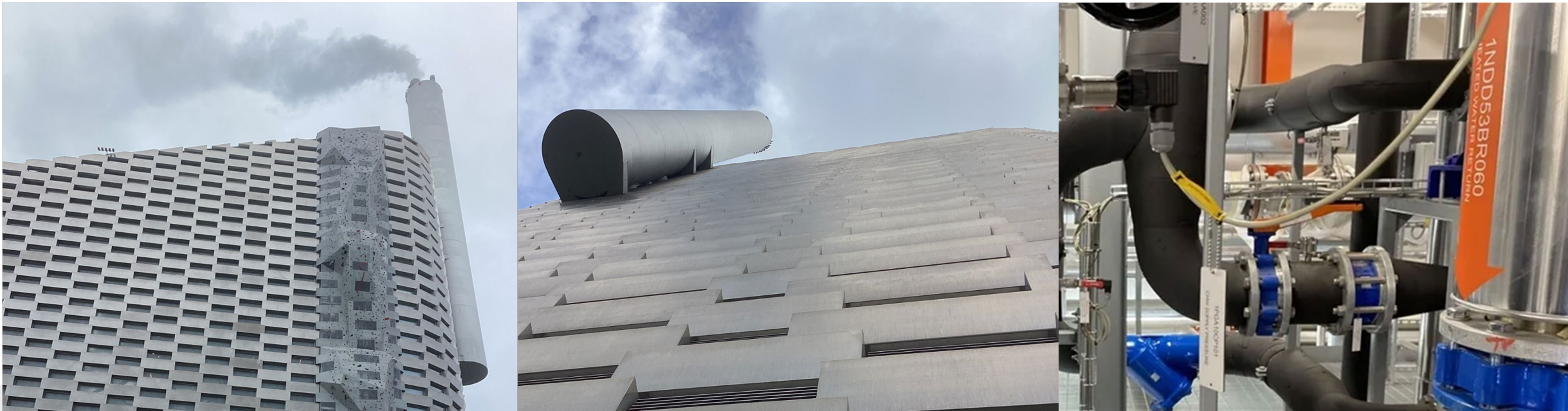
Amager Resource Centre/CopenHill, Copenhagen
