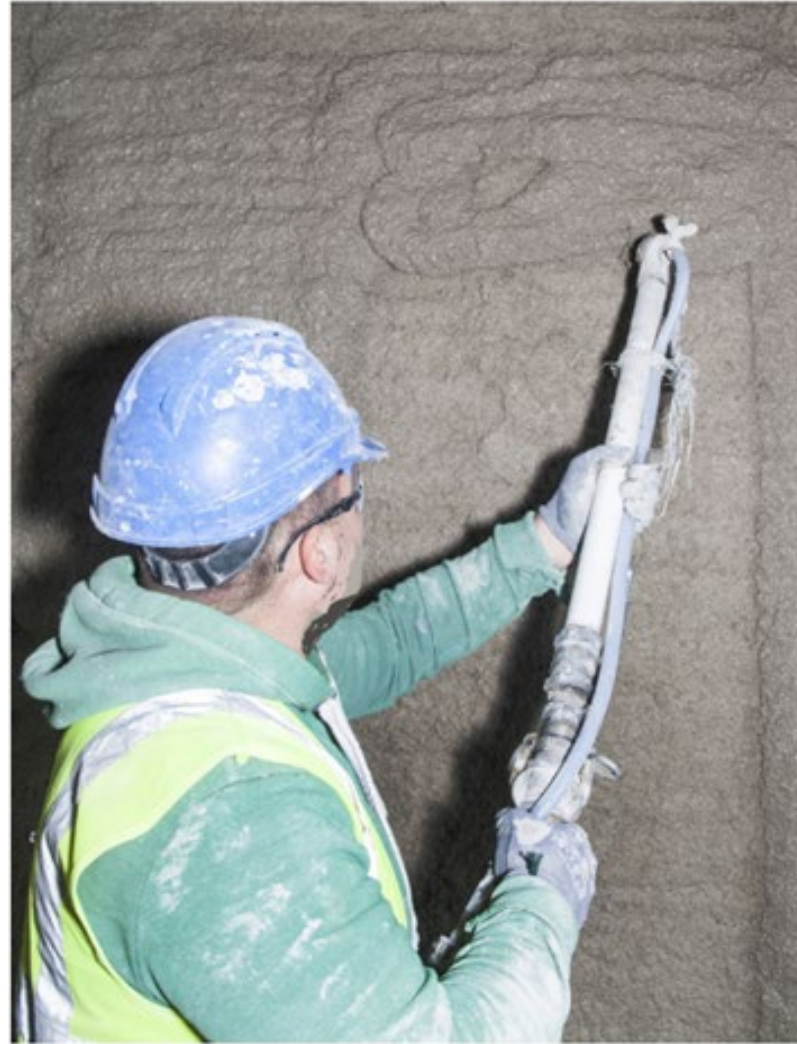
Figures 52 and 53: Insulating cork lime plaster sprayed on an uneven wall with reinforcement mesh applied below
