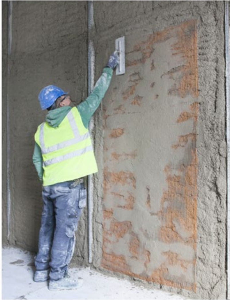
Figures 52 and 53: Insulating cork lime plaster sprayed on an uneven wall with reinforcement mesh applied below
