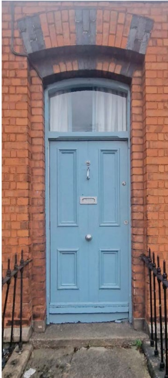
Figure 47: Aluminium draught strips can be seen to all sides of this door. Internally there is an insulated curtain
