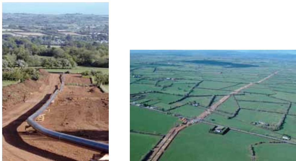
Figure 27: Cross Country Pipeline Construction in Ireland
