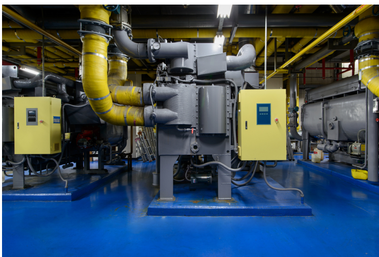
Figure 5.11: Typical absorption chiller installation
