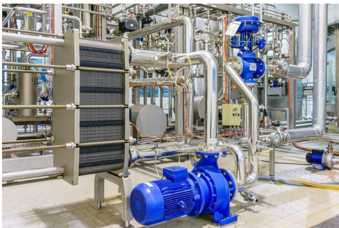
Figure 7.2: Plate heat exchanger installed with system pumps
