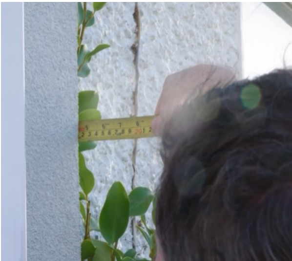
Figure 5 – EWI at boundary with adjoining house
