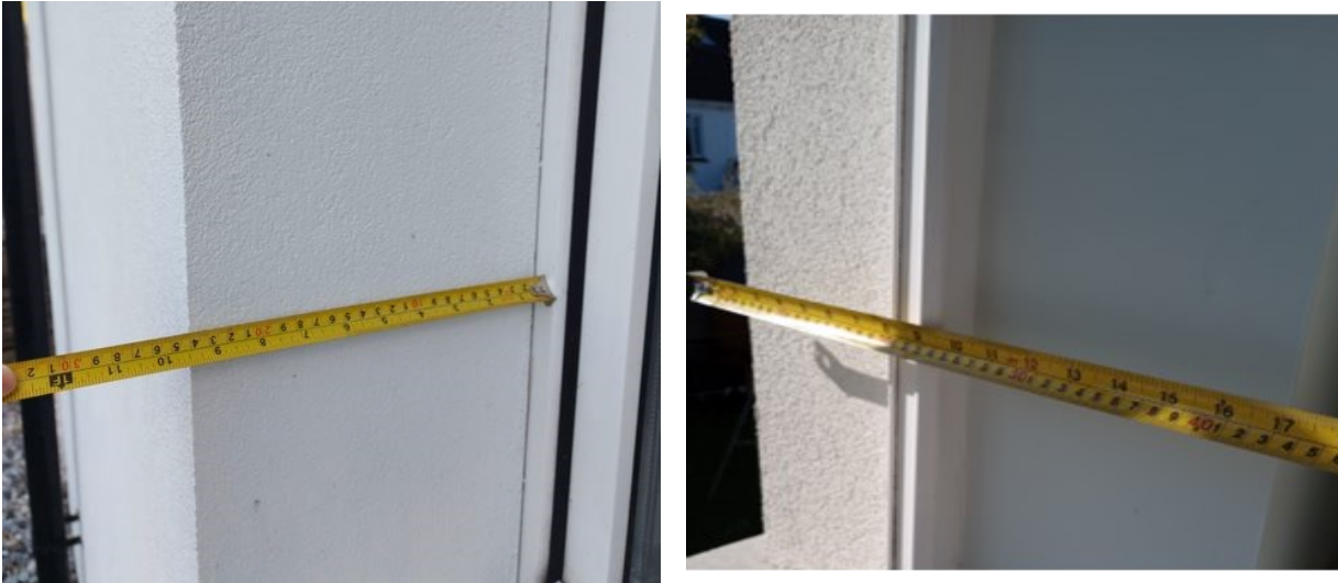
Figure 3 – Large exterior reveal depth
