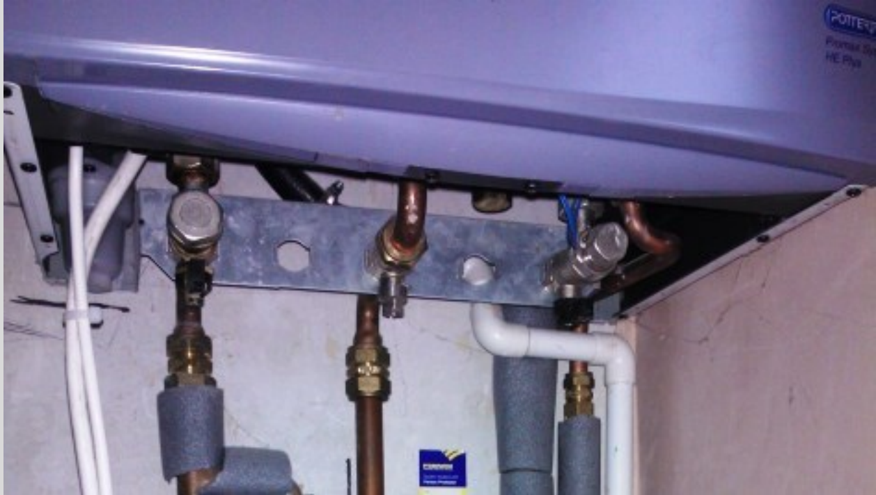
Sample image of condensate drain on a gas boiler
