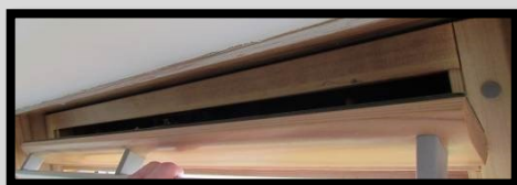
Roof window vent open
