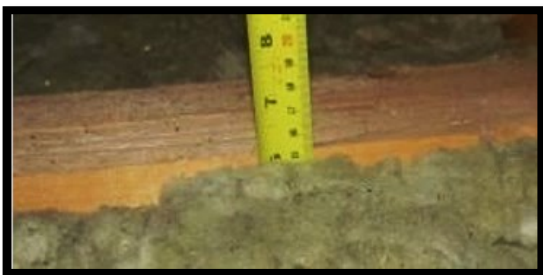
Figure 6.1: Measuring roof insulation thickness
