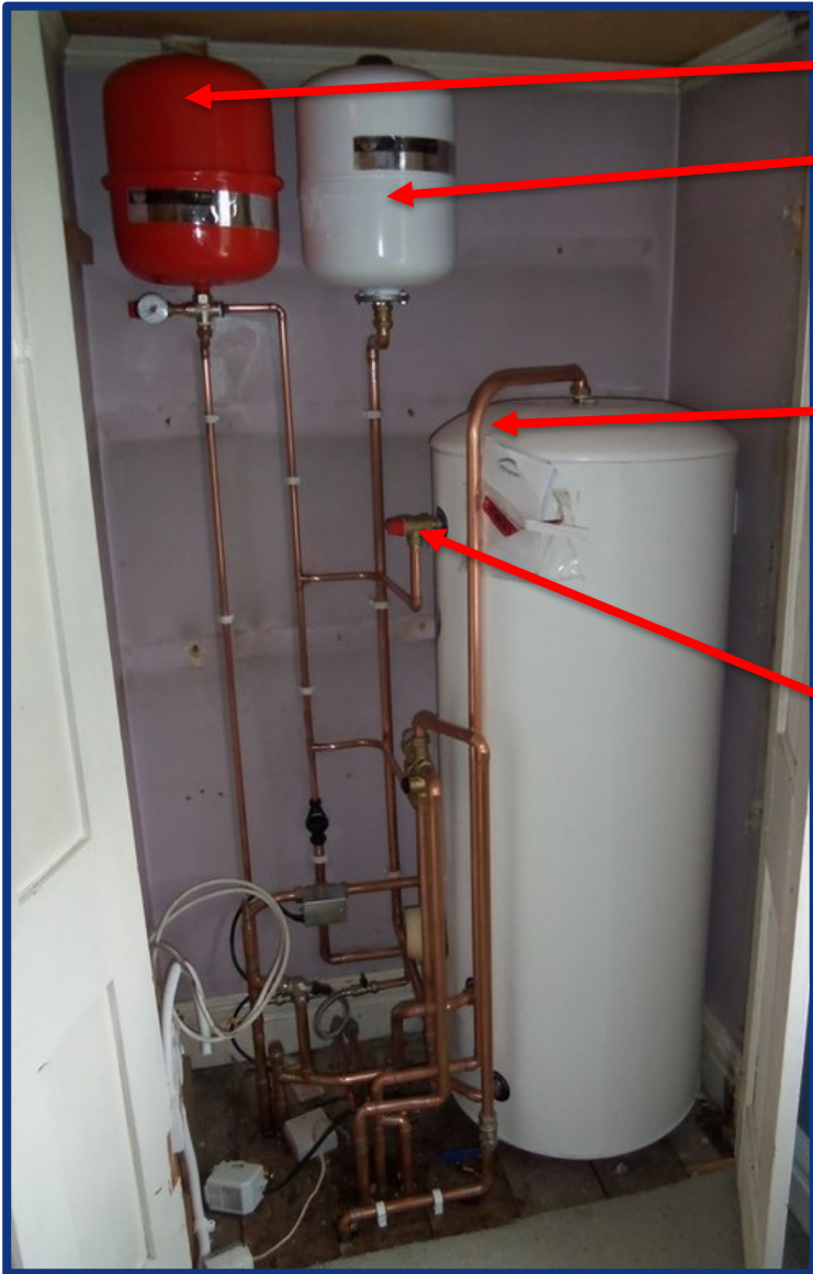
Figure 8.6 – An unvented hot water cylinder
