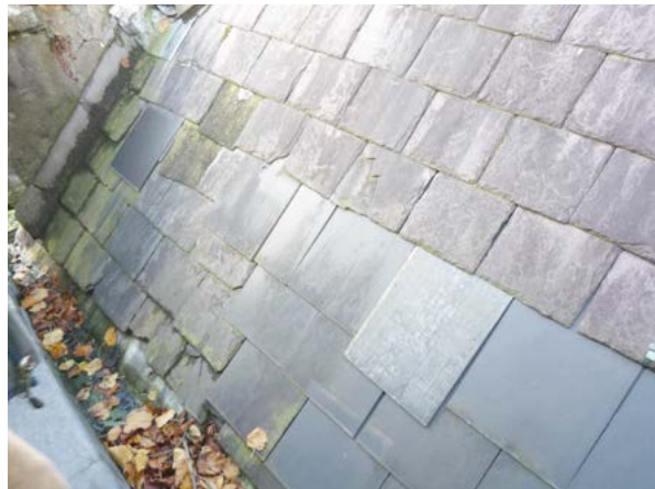
Figures 19, 20, 21: Examples of where asbestos can be found in a traditional building – panels of corrugated roof sheeting, floor tiles and roof tiles
