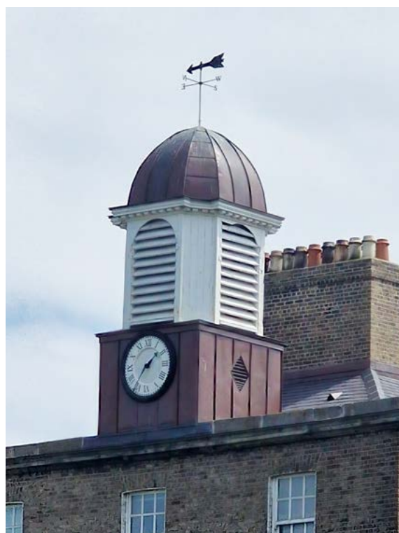
Figure 60: Copper-covered dome over louvred timber vent
