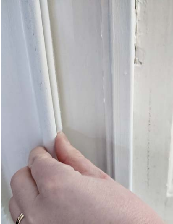
Figure 49: Discreet draught-proofing brush on a historic window
