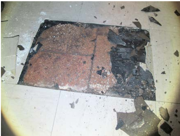
Figures 19, 20, 21: Examples of where asbestos can be found in a traditional building – panels of corrugated roof sheeting, floor tiles and roof tiles
