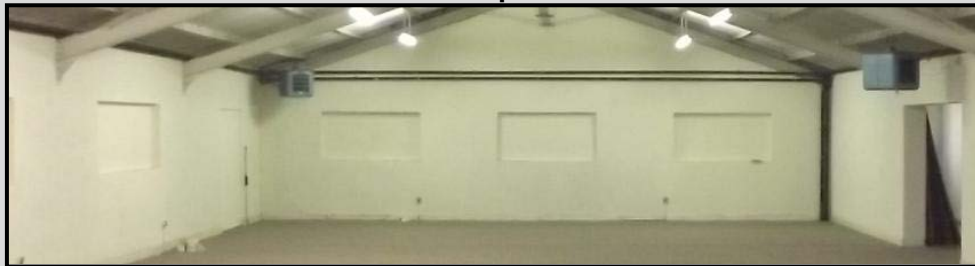
Windows slabbed over with plasterboard
