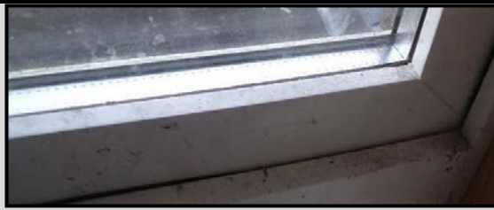
Aluminium frame, double glazed in 1970's building
