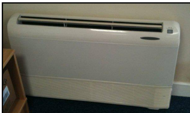
Floor mounted indoor unit
