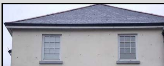
1940’s built offices
