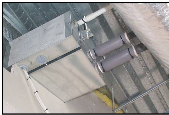
Concealed above ceiling indoor unit
