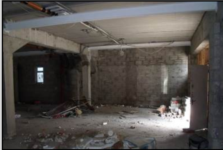
Shell and Core, no HVAC or lighting
