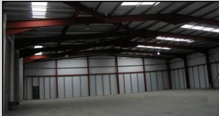
Completed warehouse zone, no HVAC, full lighting
