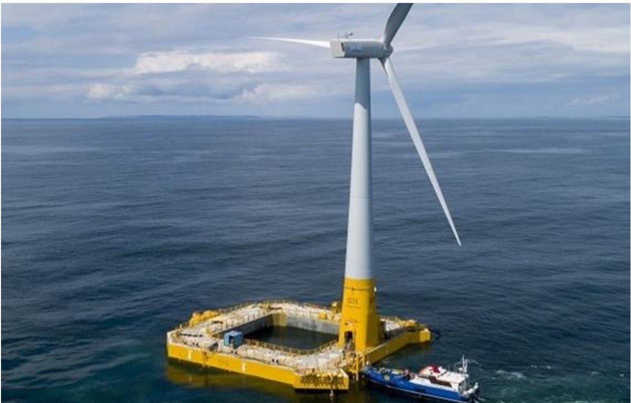
Figure 12: A concrete barge design, featuring a moonpool. Image courtesy of BW Ideol. All rights reserved
