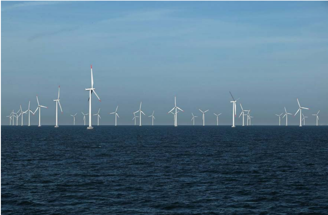
Figure 13: The Nysted offshore wind farm consisting of 72 x 2.3 MW Bonus wind turbines. Ref [17].
