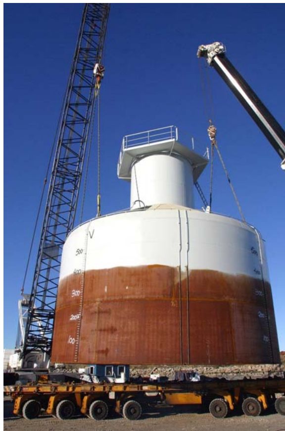
Figure 17: The bucket foundation for the Frederikshavn test site ready for transportation. Ref [13].
