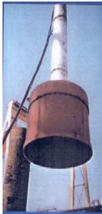
A typical pile-driving ram.
