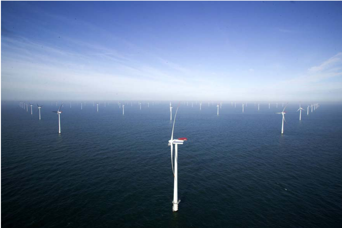
Figure 12: The 160 MW wind farm at Horns Rev consisting of 80 x 2 MW Vestas Turbines. Ref [16].
