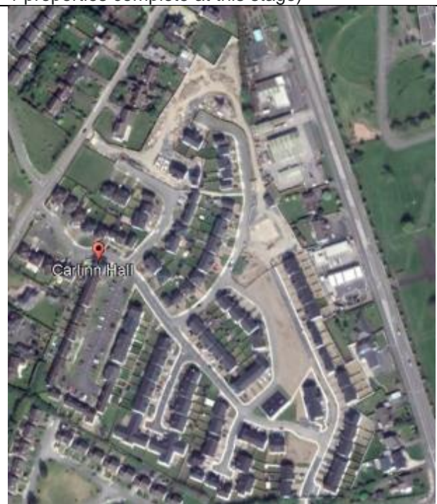
2019 – all phases of house building complete
