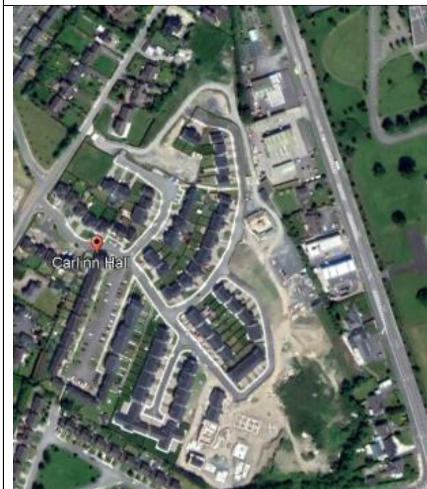
2017 – construction of phases 2-3 underway
