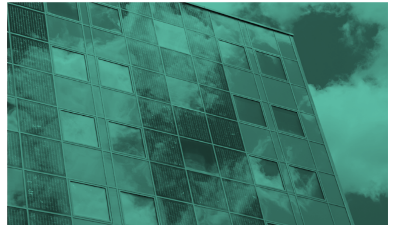
Figure 17: Solar PV Façade
